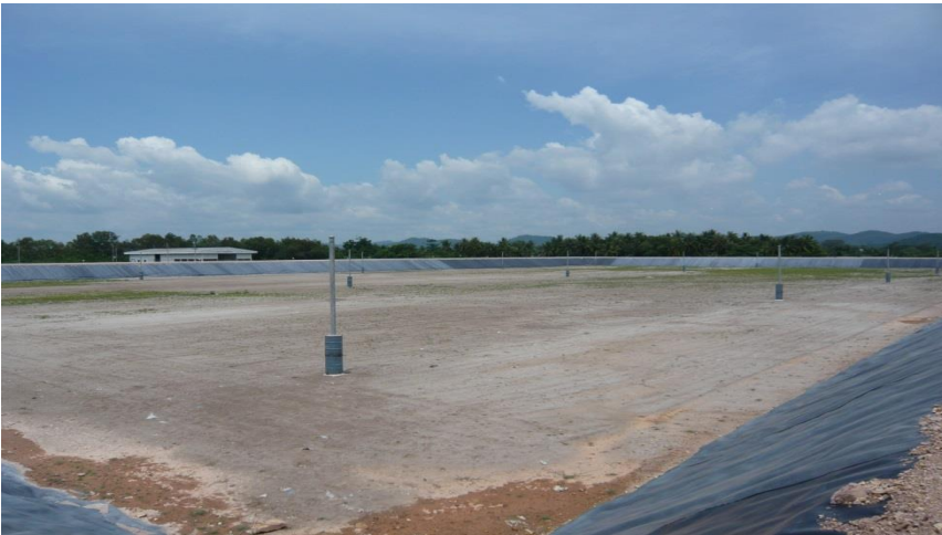
Sanitary landfill 74 sites
